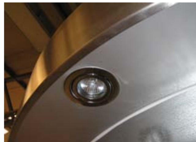
halogen illumination in stainless steel roof
