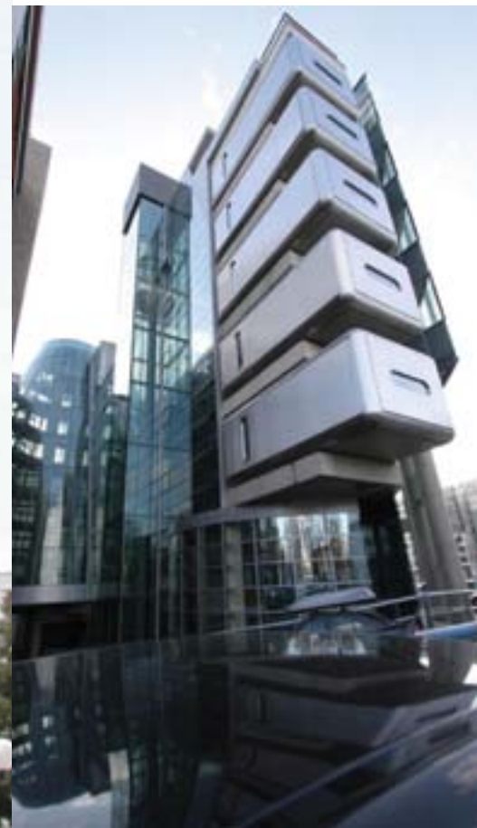
▼ prefabricated sanitary modules in new building of Croatia Insurance company in Zagreb
